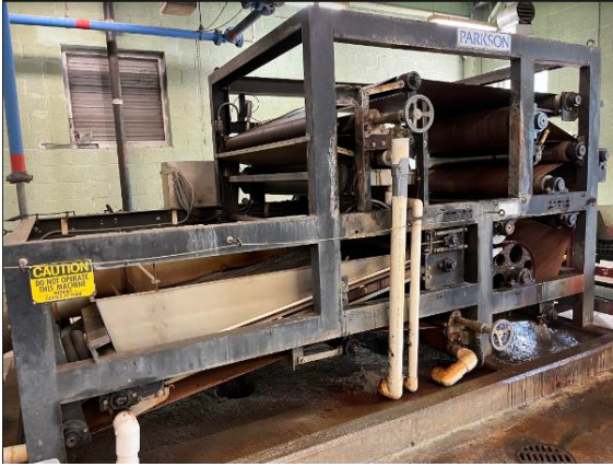
The Belt Filter Press: one of our original apparatus amazingly still in daily operation.
